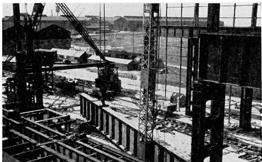
Fig. 10. 100-ton welded girder being lifted by a derrick crane and a derrick mast
