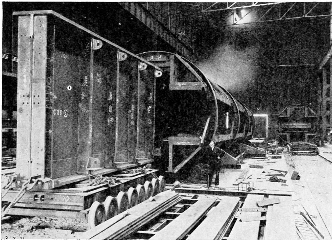
**Fig. 8.** Welded girder leaving manipulator. Second manipulator in the background
