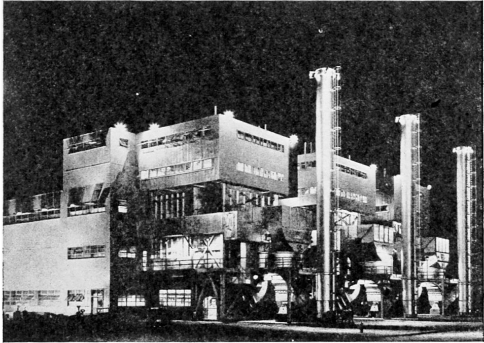
Fig. 14. Electric power plant. Light-gauge steel wall, floor, and roof panels on heavy steel frame (Detroit Steel Products Co.)
