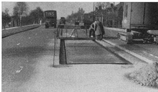
Fig. 2. Panels in Position Prior to Surfacing.
