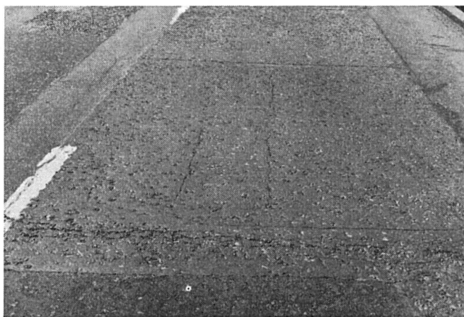
Fig. 8. General View of Bridge Panels After 2 \frac{1}{2} yr. with 1-in. Surfacing in Foreground. Note the Pronounced Cracks Over the Three Central Stiffeners and Incipient Cracks Over the Outer Stiffeners.
