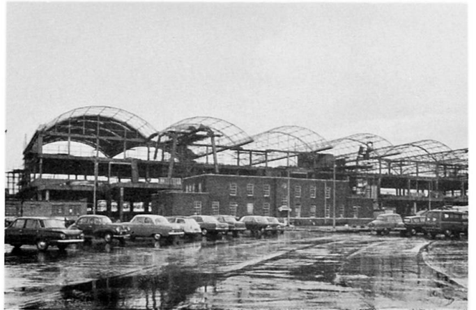
Fig. 8. The external view of seven barrel vaults built for the Port of London Authority
