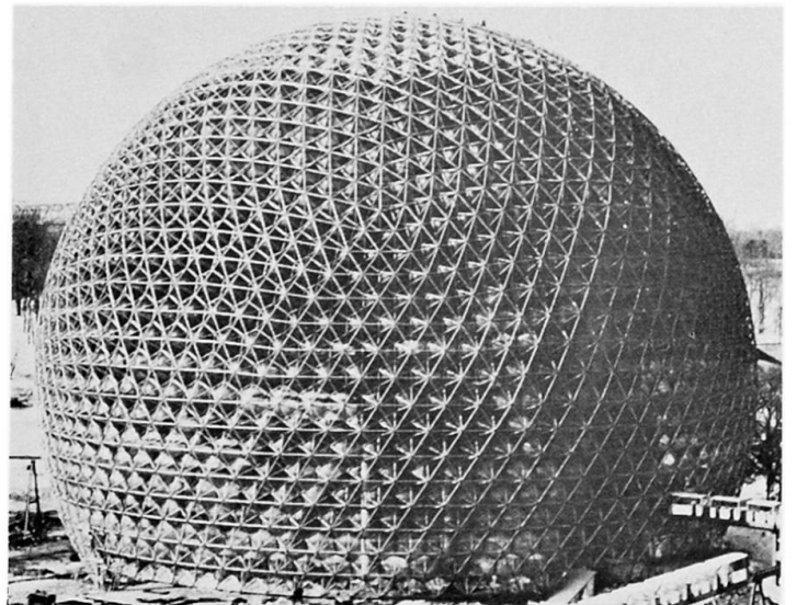
Fig. 10. Geodesic steel dome erected for the American Pavilion at Expo '67
