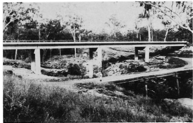
Figure 4 Submersible bridge replacing lower timber bridge
