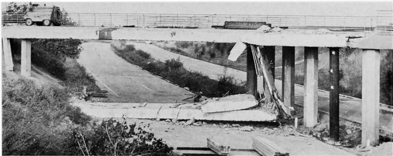
Fig. 7. The collapsed slab strip.
