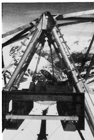
Fig. 6 Head of intermediate pylon
