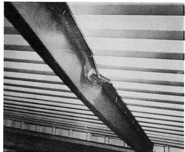
Fig.3 Buckled Z-purlin.
