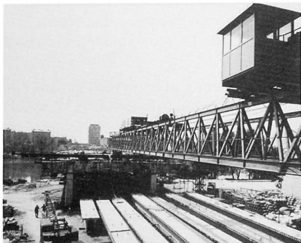
Fig. 11: Beams during grouting at the construction site.
