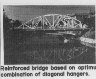
Reinforced bridge based on optimum combination of diagonal hangers.
