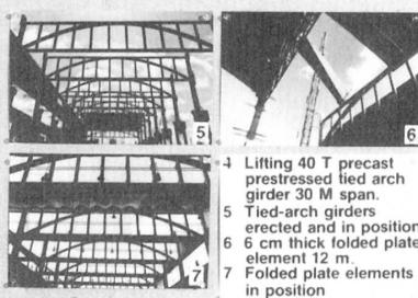
4 Lifting 40 T precast prestressed tied arch girder 30 M span.
