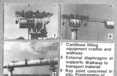
7 Cantilever lifting equipment cradles and walkway
