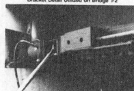
Tendon Arrangement and Bracket Detail Utilized on Bridge #2
