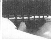
AGUASABON R. Bridge New transversely laminated, prestressed wood. Segmental Construction. Terrace Bay, Ontario 1983.
