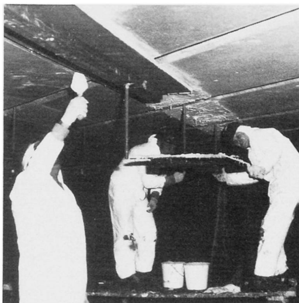
Fig. 3 Bonding of Steel Plates
