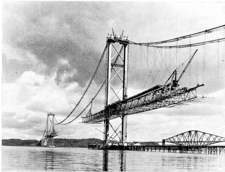
Fig. 8. A view during erection of suspended structure. Note temporary upward deflection of steelwork.
