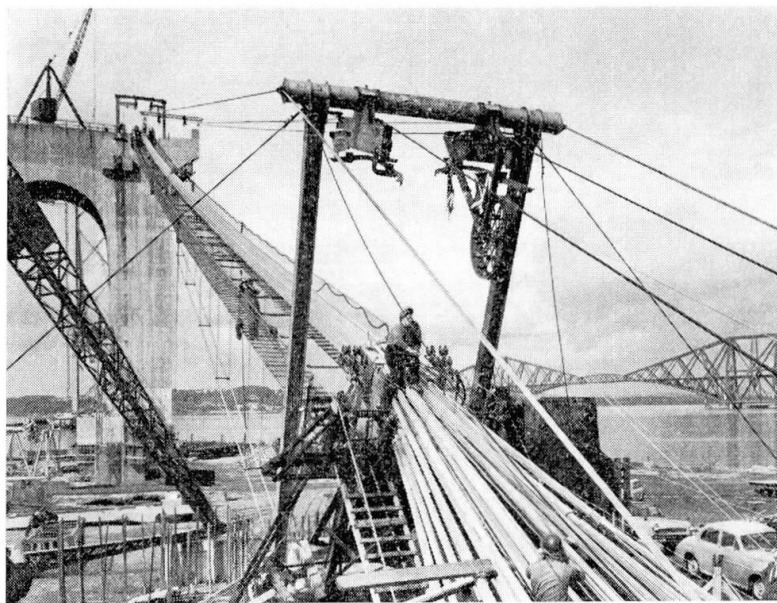
Fig. 5. Cable spinning nearly completed — the last spinning wheel leaving the South anchorage.
