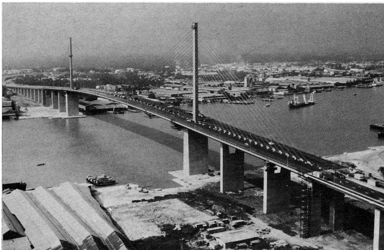
The newly completed Rama IX Cable-Stayed Bridge over Chao Phraya River in Bangkok, having a span length of 450 meters, the longest among all single-plane cable-stayed bridges.
