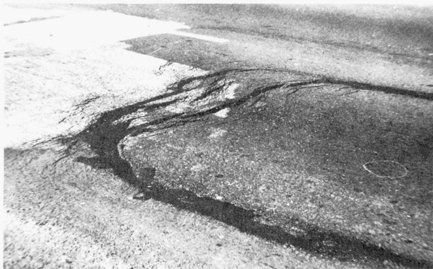
FIGURE 3. MODE OF FAILURE DUE TO DEBONDING OF THE AC PAVEMENT ON THE ULATIS CREEK BRIDGE AFTER ONLY A FEW MONTHS IN SERVICE
