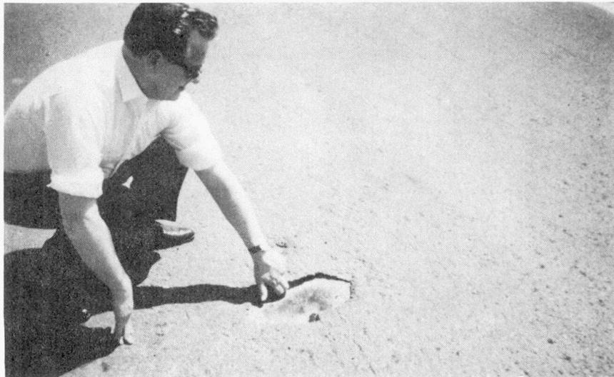
FIGRE 5. BREAKOUT OF WEARING COURSE OVER SPLICE PLATE ON CONCORDIA BRIDGE AFTER TWO YEARS OF SERVICE
