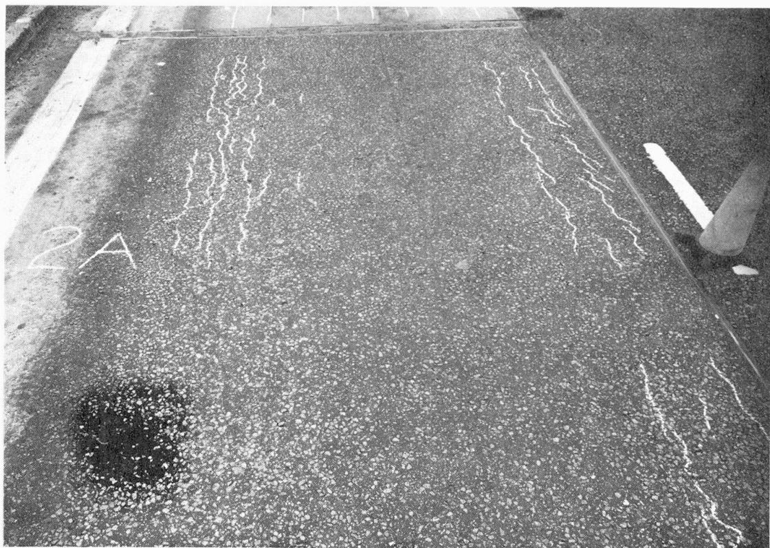
FIG. 4 CRACKING ON ROLLED ASPHALT OVER GRITTED EPOXY RESIN, NOVEMBER, 1967
