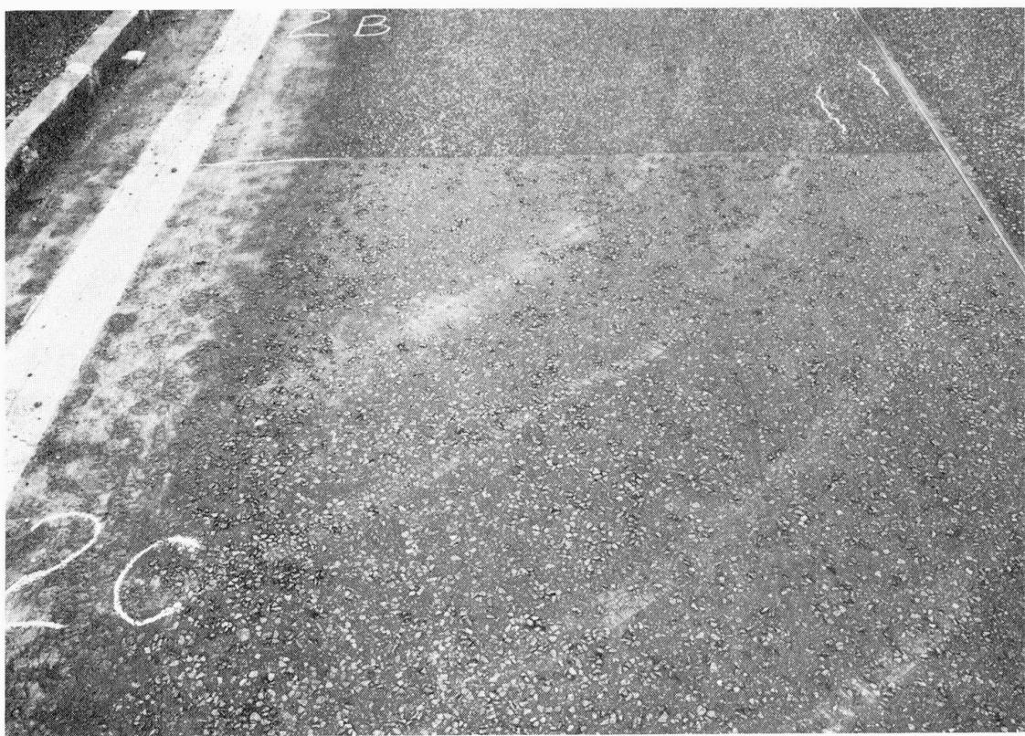
FIG. 7 MASTIC ASPHALT ON FILLED RUBBER BITUMEN, NOVEMBER, 1967
