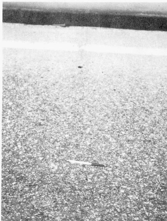
FIGURE 2. EVIDENCE OF A TRANSVERSE CRACK FORMING OVER THE SPLICE
