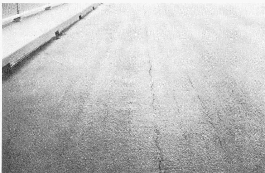
FIGURE 4. LONGITUDINAL CRACKS IN THE ACPAVEMENT ON THE CONCORDIA BRIDGE AFTER TWO YEARS IN SERVICE
