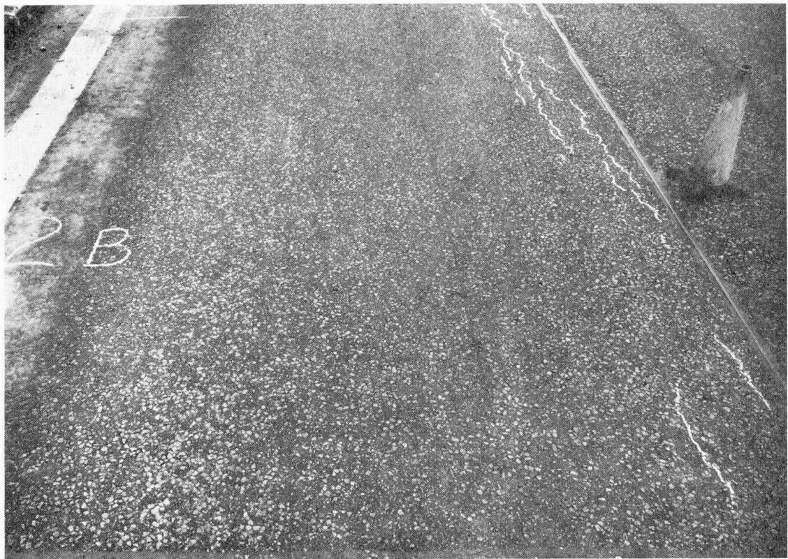
FIG. 6 CRACKING IN ROLLED ASPHALT ON FILLED RUBBER BITUMEN, NOVEMBER, 1967
