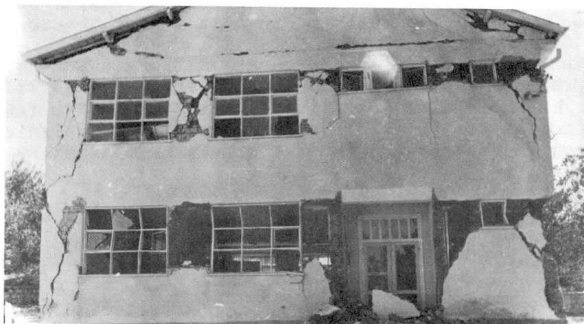
Figure-5 Typical Failure of Brick Masonry
