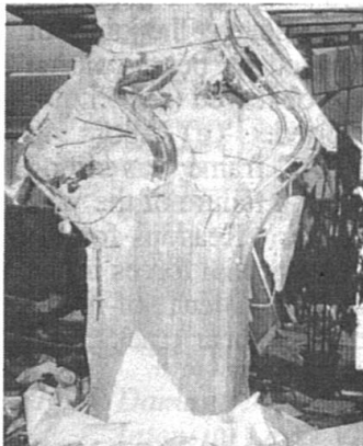
Photo. 2 Collapsed Column in Shear
