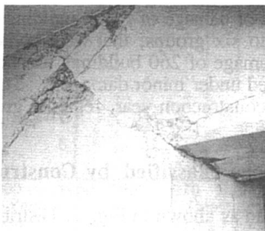
Photo. 6 Damage of Beam-Column Connection
