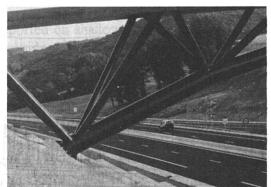
It was decided to fill the bottom parts of the arch with concrete to improve the structure's resistance to collisions with outsize vehicles.
