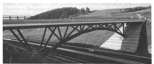
The bridge carries a 11 metres wide roadway. Its total length is 86 metres between the end support axes. It is designed to give the passage to exceptionally heavy 110-ton trucks.
