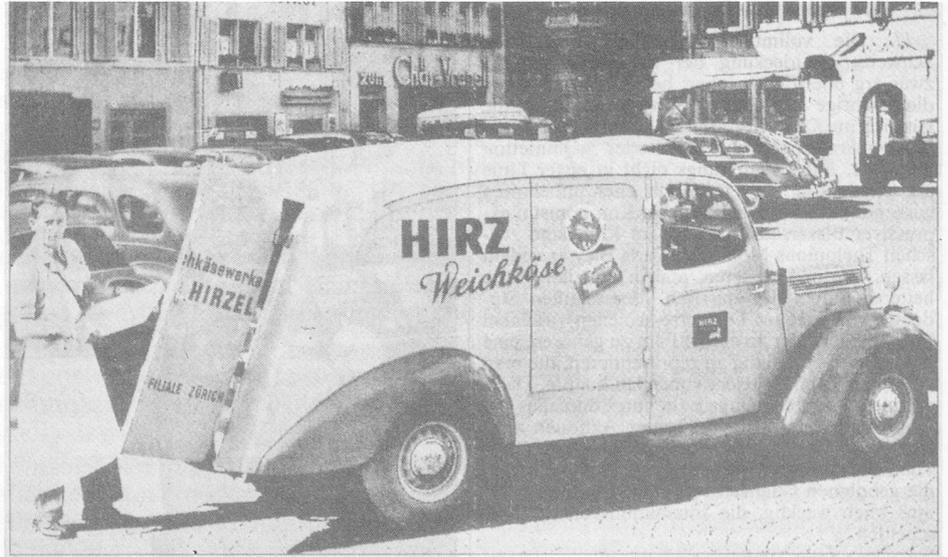
Delivery of fresh produces in the "old days" where the products were kept literally on ice inside the van by means of the then famous ice bars at the time where refrigerated trucks were still unknown.
