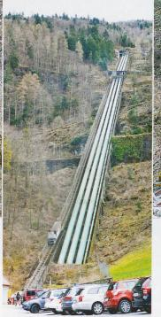
ABOVE: Just above the valley station next to the 3 pressure pipes leading to the Power Station.
