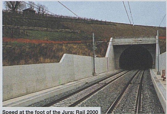
Speed at the foot of the Jura: Rail 2000 tunnel near Gorgier NE
