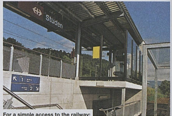
For a simple access to the railway: customer-friendly stopping points
