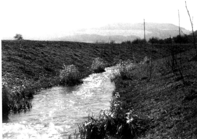
Left: Embankment protection with fascine, open fascine layer combinations (1 year after planting).
