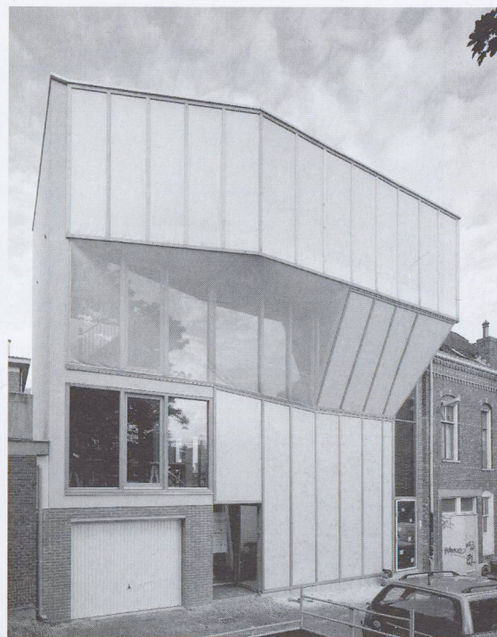
Blue Moon – Achter de Barakken, Space Group Architects
