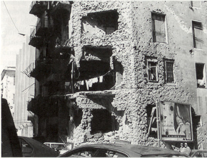
Severe damage was done to these buildings in Beirut, Lebanon, after a massive air attack by the Israeli Air Force.
