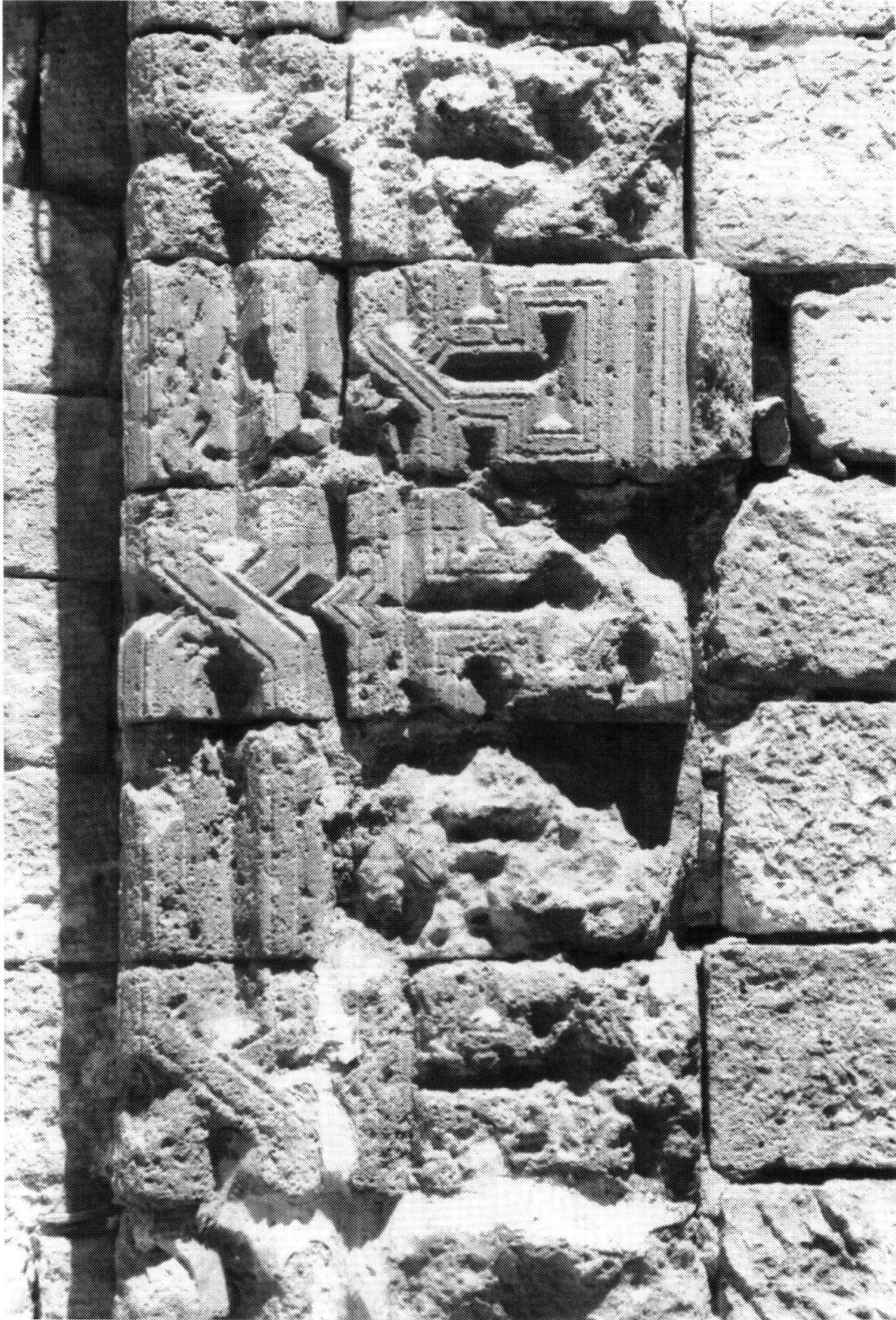
Figure 9: Mardin: Madrasa Šahīdiyya, north wall of courtyard, rest of pillar.
