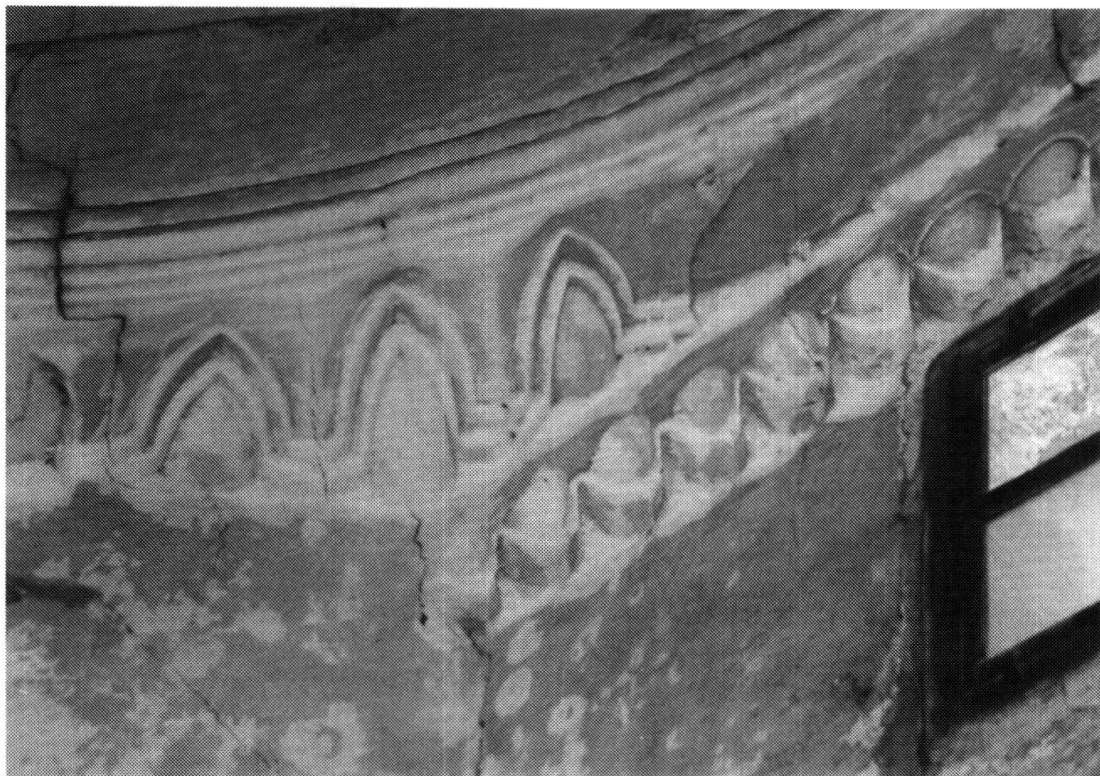
Figure 3: Mardin: Madrasa Sittī Raḍaviyya, mausoleum's tambour, wall south.
