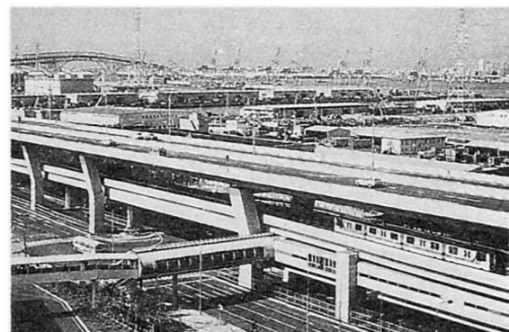
Fig. 9 Modern expressway/trunk combination: Osaka - Wangan Route
