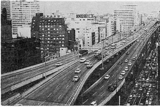
Fig. 4 Semba Rooftop Expressway: Osaka
