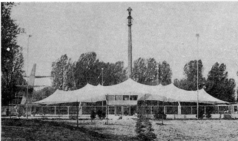
Fig. 3 Swimming Arena Düsseldorf Tractor in base position, docked to the anchorage.
