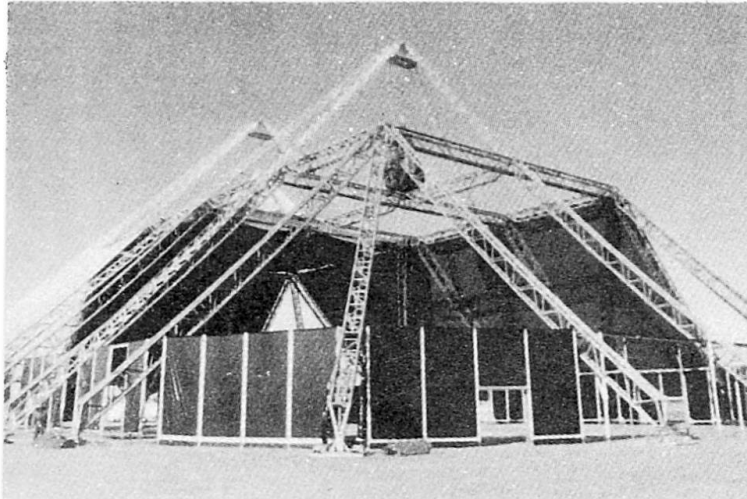
Figure 7 - Erection: installing fabric
