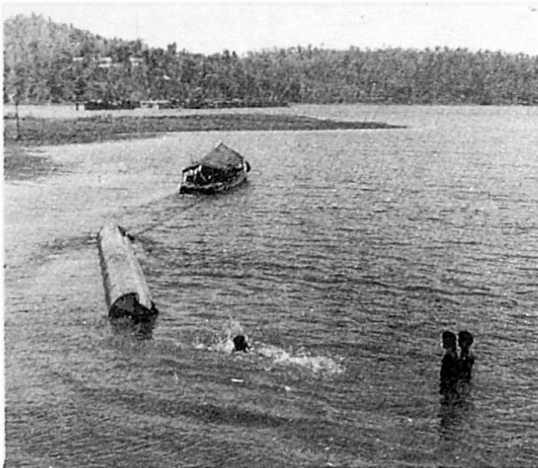
Photo.3 1000mm diameter casing being towed to site
