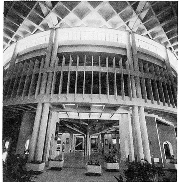
Fig.3 View of Assembly Hall from podium level
