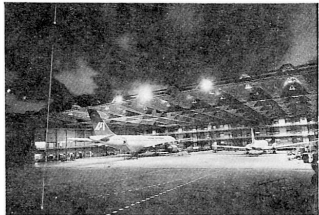
Fig.21 Indian Airlines Hangar, Bombay
