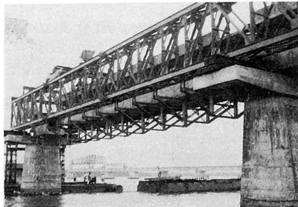
Fig.12 Assembly Truss
