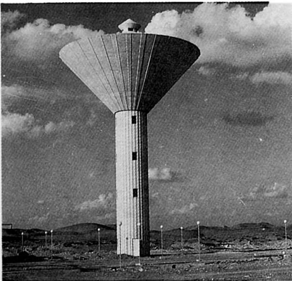
Fig.33 Haza Al Maqam reservoir, U.A.E.
