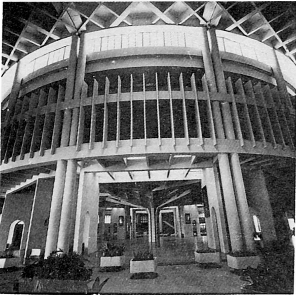
Fig.24 Assembly hall, Gandhinagar
