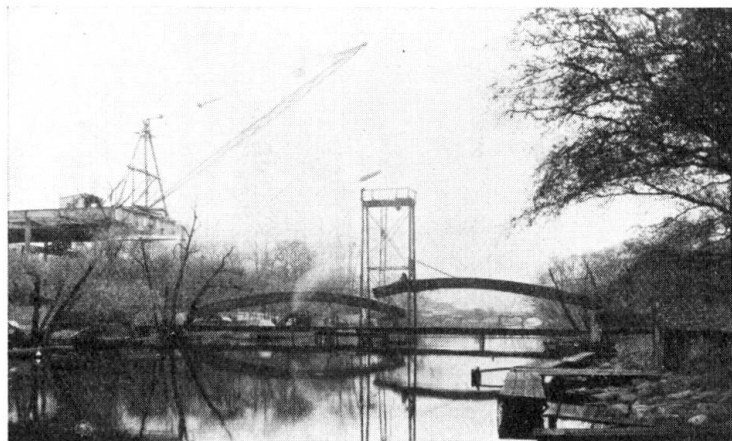
Fig. 14. Pålssund Bridge. Erecting the arches.
