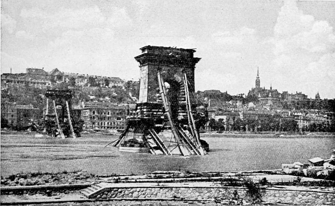
Fig. 4. View of the blown up « Chain-bridge » Budapest.
