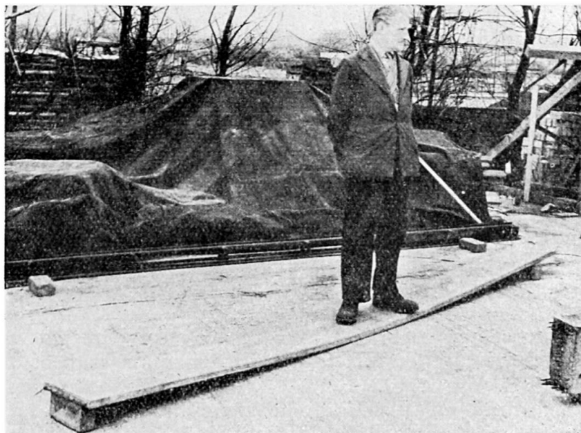
Fig. 3. Prestressed concrete plank 1 \frac{1}{4} " thick, 12 ft span.
