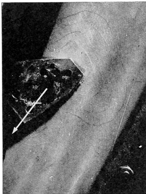
Fig. 9. Application of the brittle coating method to the determination of the isostatics in a spillway guide wall
