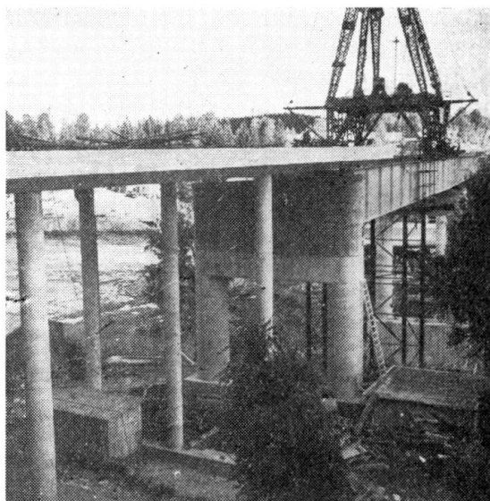
FIG. 13. Concrete viaduct at Bergeforsen, Sweden
