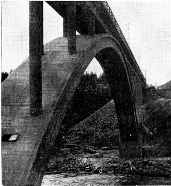
FIG. 1. Railway bridge over the river Vindelälven in North Sweden
