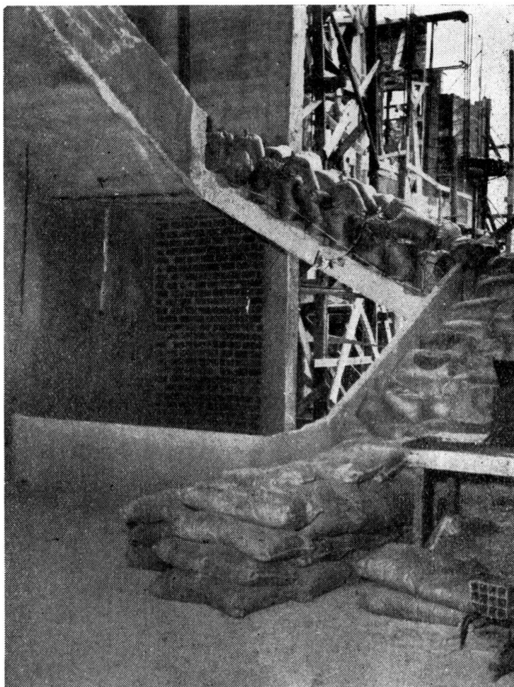
FIG. 8. Application of the uniform load
