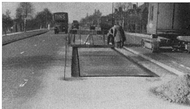
Fig. 2. Panels in Position Prior to Surfacing.
