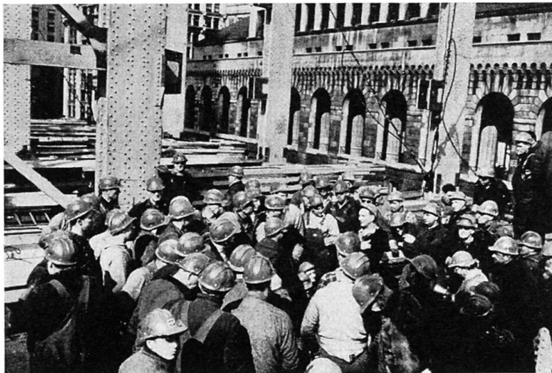
Fig. 17. Safety meetings should be held regularly, and safe operations result in efficient and economical production.
