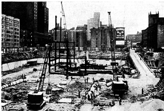
Fig. 1. Guy derrick consists essentially of boom, mast, falls for raising or lowering boom and load, and guys to hold mast upright.
