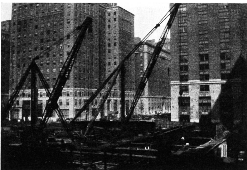
Fig. 14. Stiffleg derricks are sometimes used as travelers to erect heavy steel below street level, then setting up guy derricks for the upper, lighter structure.
