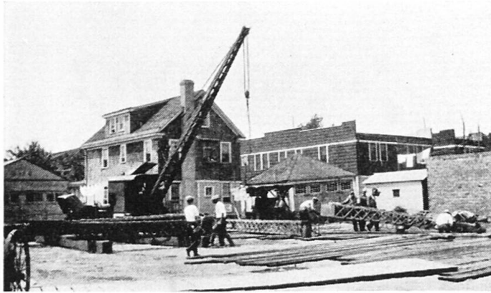
Fig. 4. Use of a crane is advisable to unload tools and equipment, and then to assemble and set up guy derrick.
