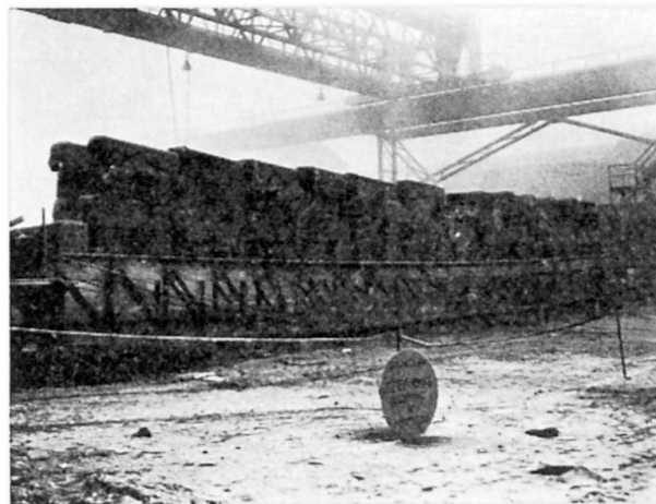
Fig. 1. 1st Full Scale Test. View of Girders at Failure.
