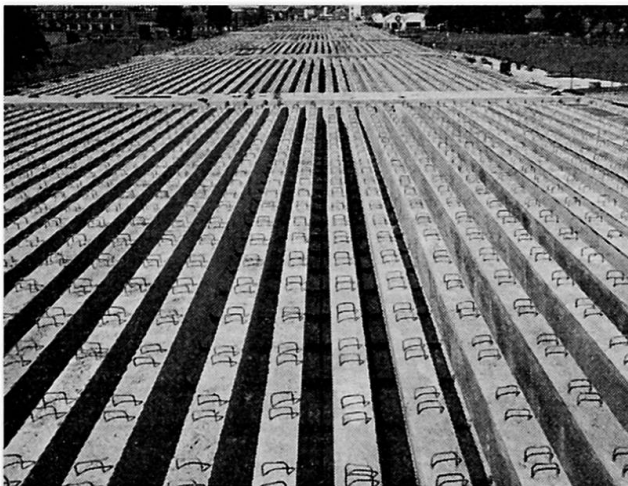
Fig. 7. Prestressed bridge beams in the Chiswick-Langley motorway.
