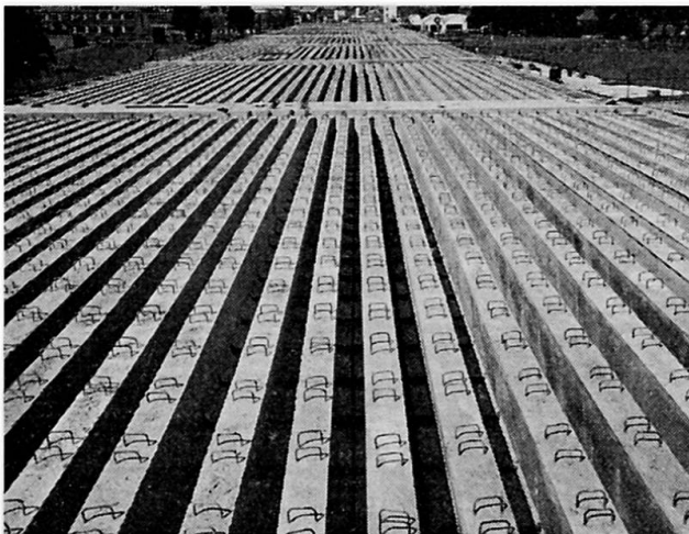
Fig. 7. Prestressed bridge beams in the Chiswick-Langley motorway.
