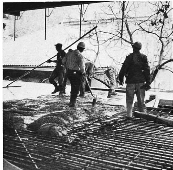
Fig. 10. Category I Form — View showing placement of concrete. (Note negative reinforcing bars.)
