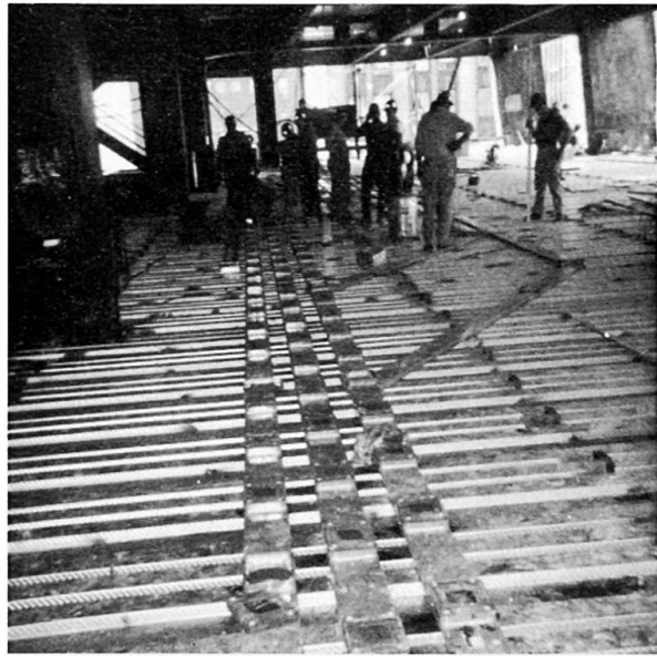
Fig. 12. Category II(b) Form – View showing raceways for wiring with uniformly spaced service fittings.
