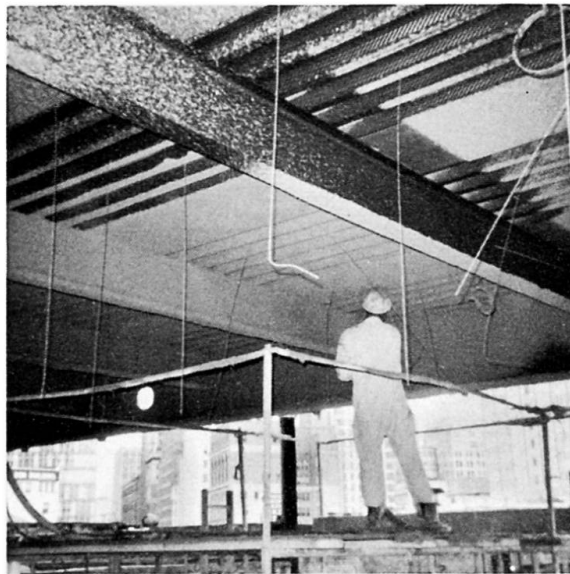
Fig. 14. Category II(b) Form – Application of spray-on fireproofing.
