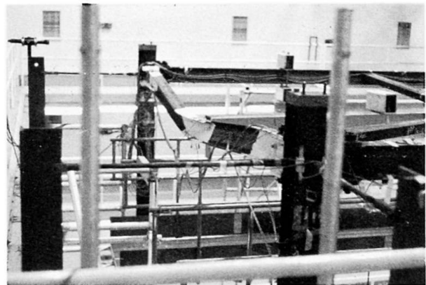
Fig. 5 - Major-Axis Beam at Collapse
